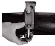
5. Housing installation
