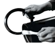
2. Lubricate gasket
