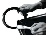
2. Lubricate gasket
